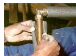
Insulating hot water pipes with foam
